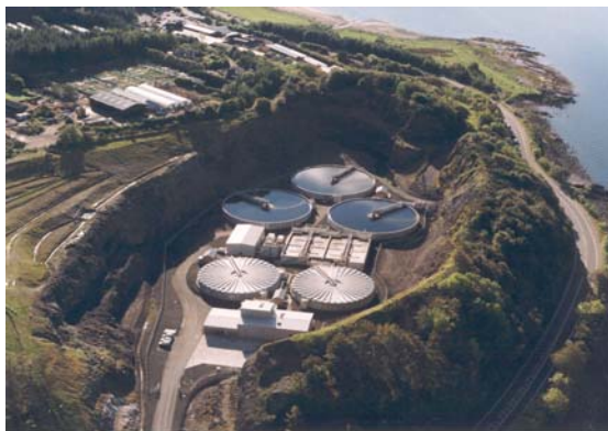
Waste Water Treatment
